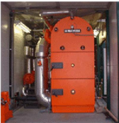
**Figure 6.7. This Austrian-built Stirling engine powers a generator capable of producing 75kW of electricity. The heat output from both generator and boiler is 500kW.**
