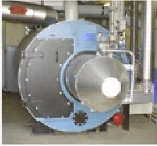
**Fig. 6.14 Retrofitted oil-fired boiler**
