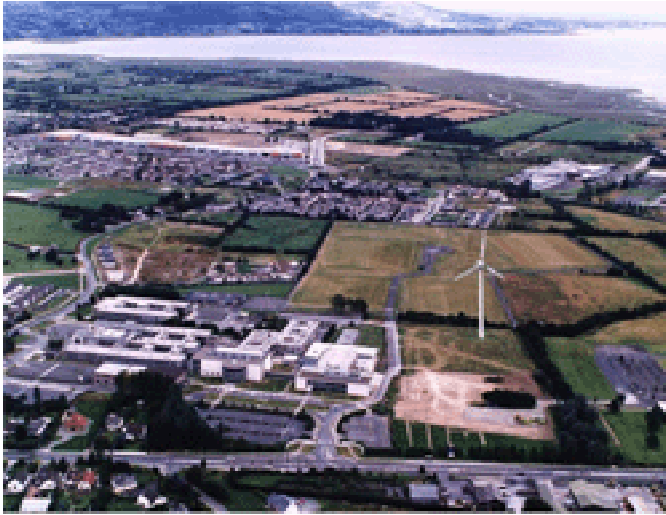
photomontage showing the Dundalk Institute of Technology campus, the turbine and the Irish Sea in the background.
